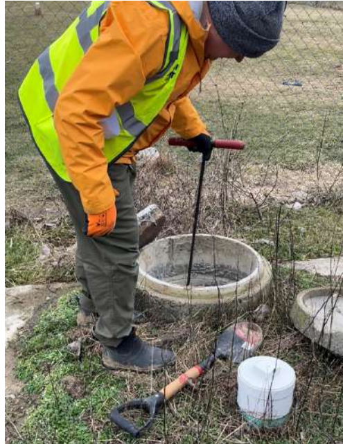
ZACHARY, REHS, PERFORMING A LEACH FIELD SEPTIC INSPECTION
